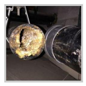
Photo provided by UC Berkeley Facility Services: Sanitary sewer pipe cross-section with build-up of FOG; the blockage narrows the pipe and restricts the volume of water that can flow through the pipe.
