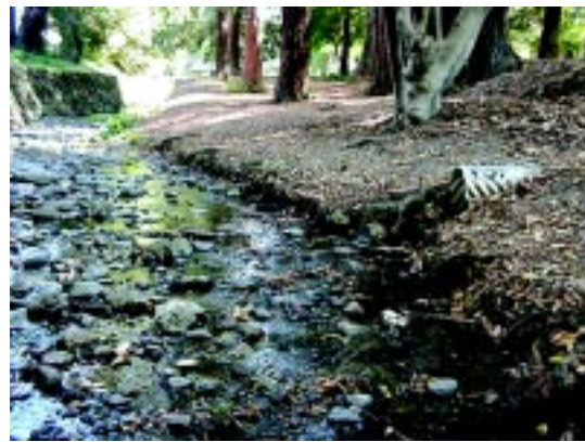
Note the pipe on the right. Discharges to the storm drain flow directly into Strawberry Creek and San Francisco Bay untreated.
